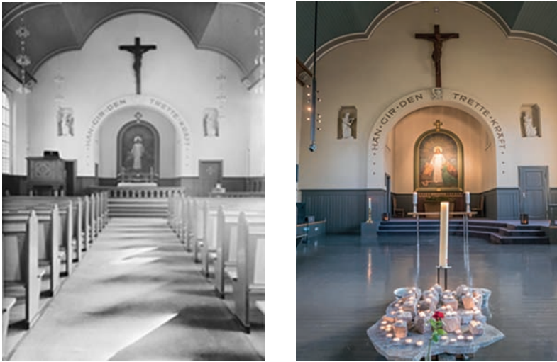
Figure 8: Pictures of Tøyen kirken, Oslo. On the left, an official picture from 1969 40 , and on the right, the same church today (Photo: Andreas Kiil).
