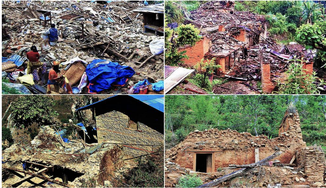
Figure 5: Physical damages of houses and assets
